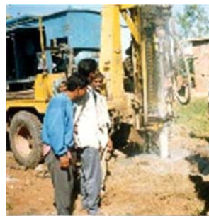
Boring a well for community drinking water
